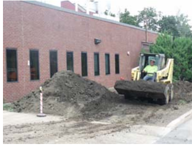
Office During Removal and Preparations
